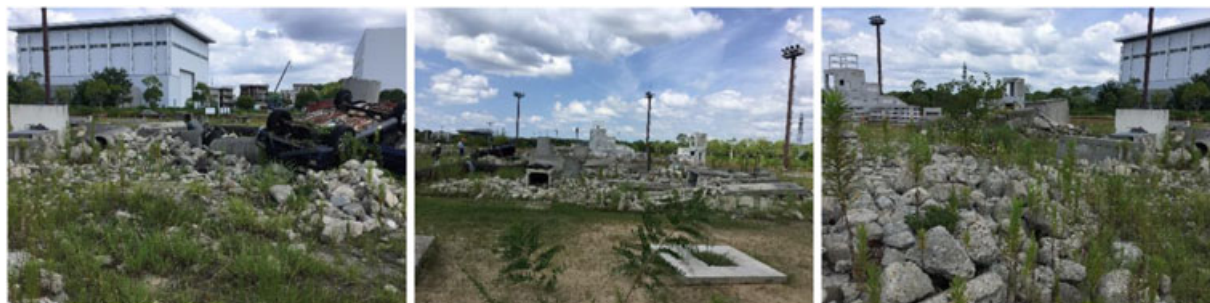
FIGURE 8 The rubble field at Hyogo Prefectural Emergency Management and Training Center [Color figure can be viewed at wileyonlinelibrary.com ]
